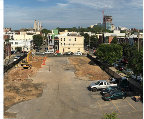
June 2016 - Construction at the Arthur Schoolyard begins.
